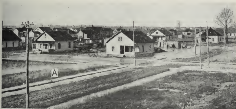
FIG. 46.—Flooded streets, broken sidewalks and foundations, and damages to plastering resulting from subsidence in Franklin County. Figure 48 shows the broken sidewalk at A. (Photo by H. I. Smith, U. S. Bureau of Mines.)
